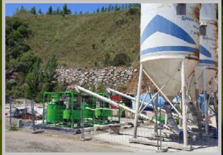
Automatic mixing plant, supplied by silos. They are located at the base of the dam.
