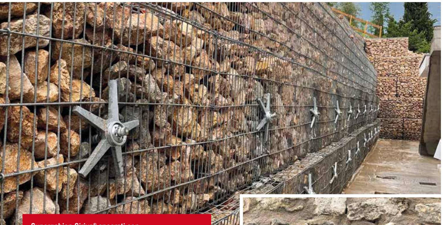
Supergabion Sirive® ancorati con barre autoperforanti e piastre Sirive® Stella Sirive® Supergabion anchored with self-drilling bars and Sirive® Star plates
